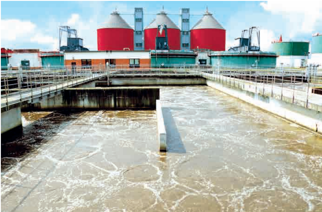
In the foreground: Water is aerated in aeration basins. In the background: Three digesters.
