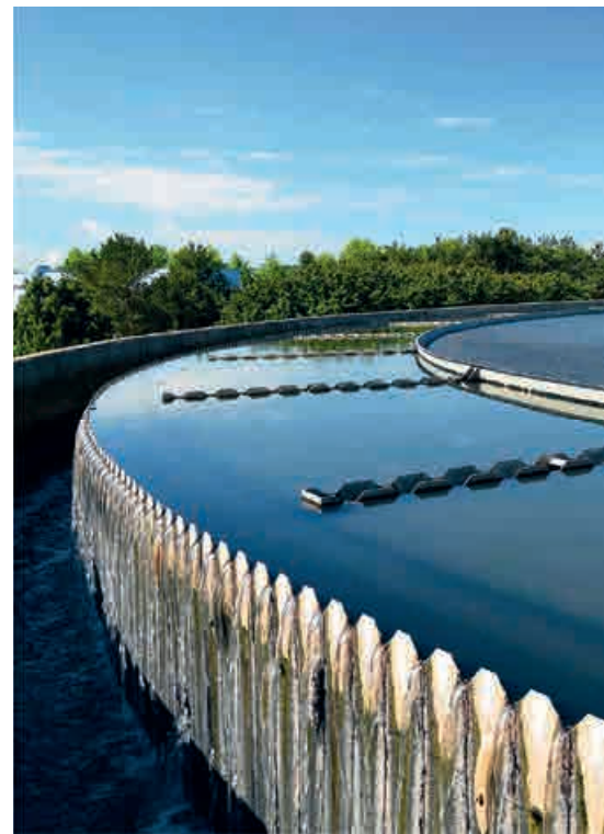
The clear, biologically purified water flows out of the secondary clarifier.
