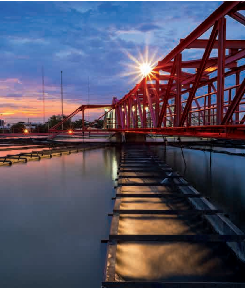
Evening atmosphere at the sewage treatment plant
